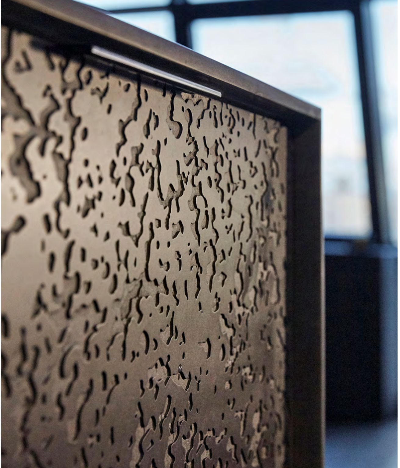
Detail of the charcoal-colored MDF kitchen millwork, textured through CNC routing, mimics the texture and warmth of the fireplace. The screen, cabinets and floor frame the white interior walls that display the owner's art collection.
